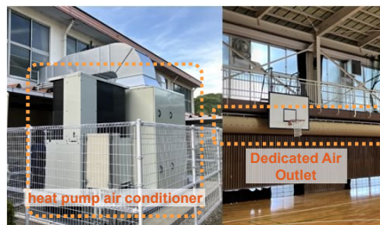
(Left) BREEZE for ARENA installation status at an elementary school in Hadano City (Right) Measurement of air conditioning effect (thermography) during BREEZE for ARENA operation
